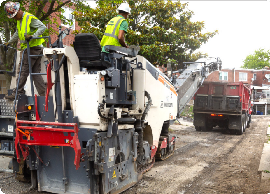
Neighborhood Driveway Repair
